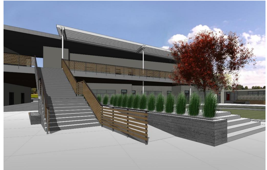
Two-story Building View from Science Courtyard
