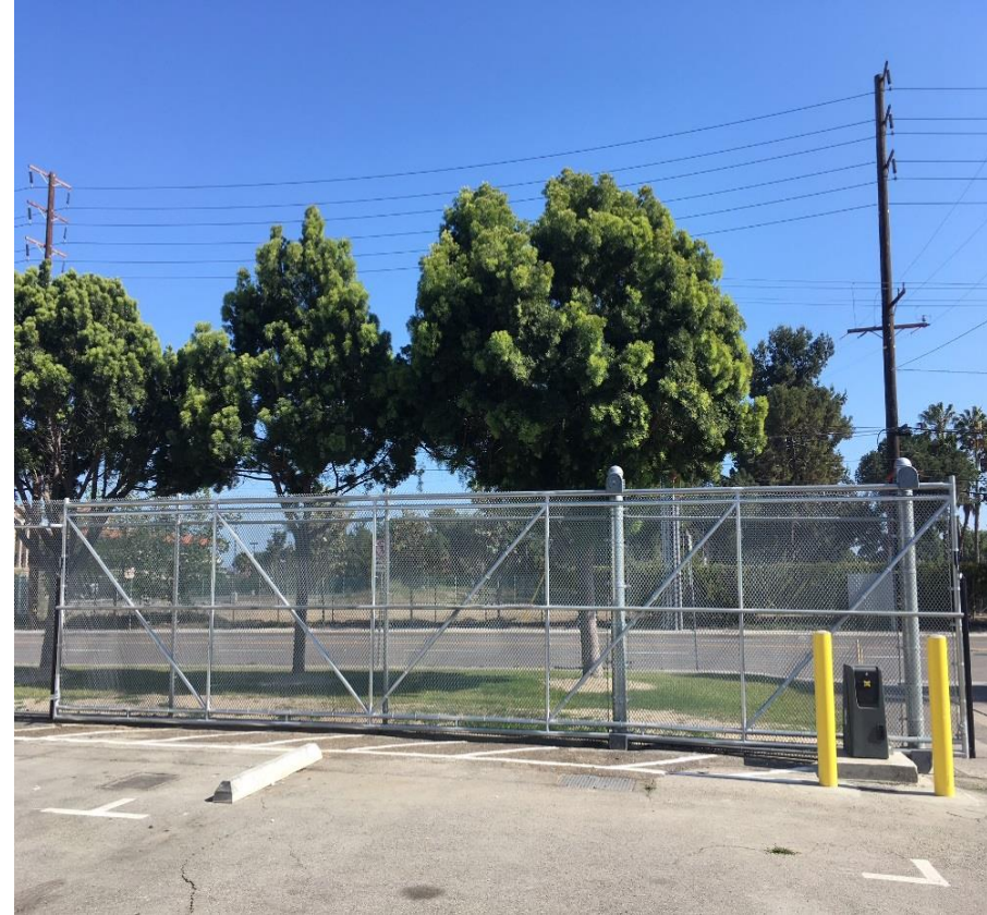
New Motorized Gate
